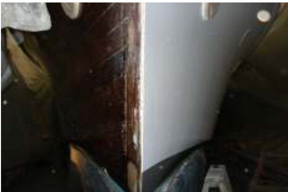
PAM is half in MAS Epoxy & half in HMG Polykote Primer
